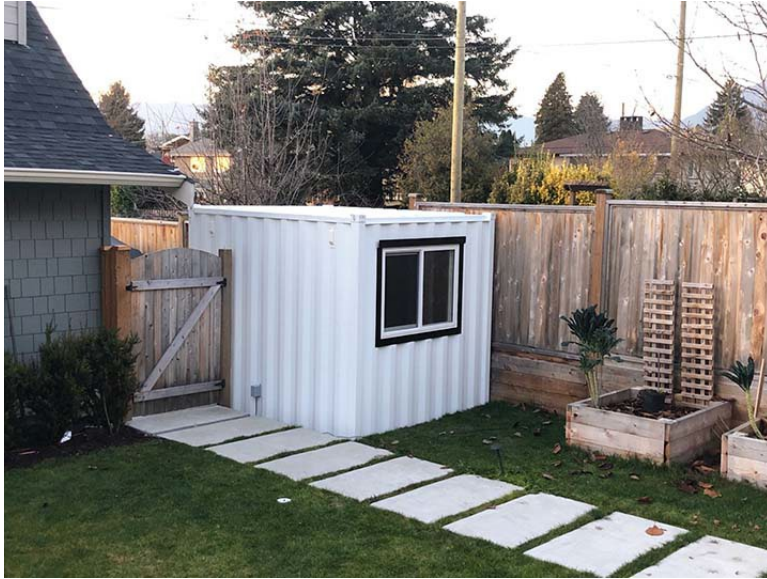
Figure G – Shipping Container
