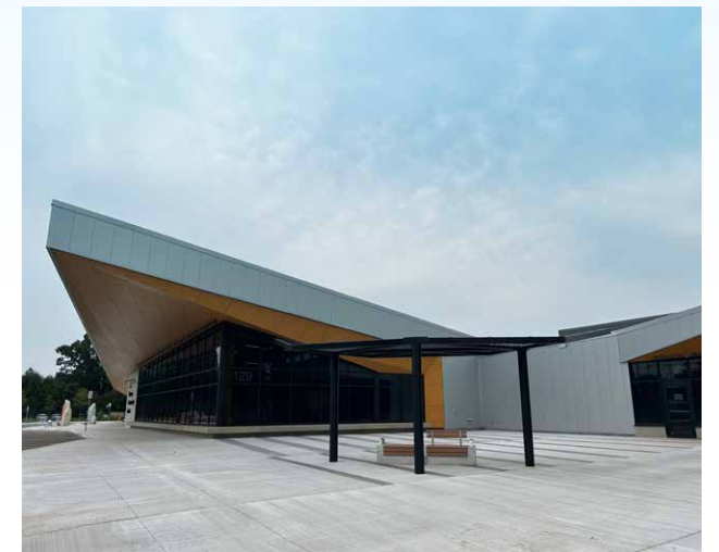
Accessible entrance at Skyway Community Centre with bench seating
