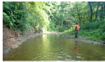
AOC 2 - erosion along valley wall toe; risk to property
