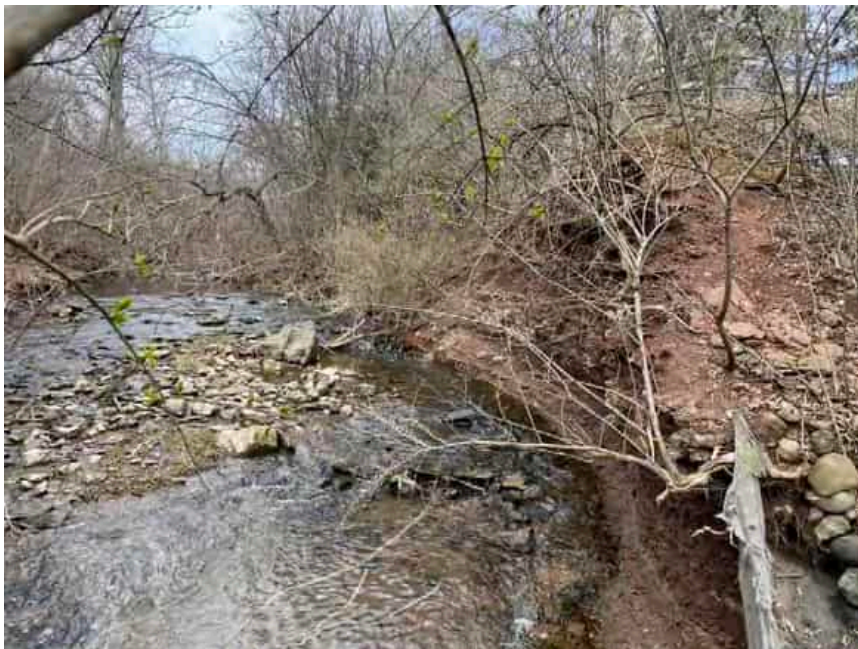
Photo 18: Bank erosion immediately upstream of stormwater outfall adjacent to the parking area of Branthaven Homes
