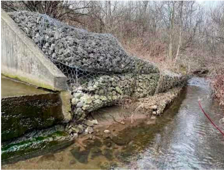
Photo 16: Gabion baskets along the east bank of reach 3
