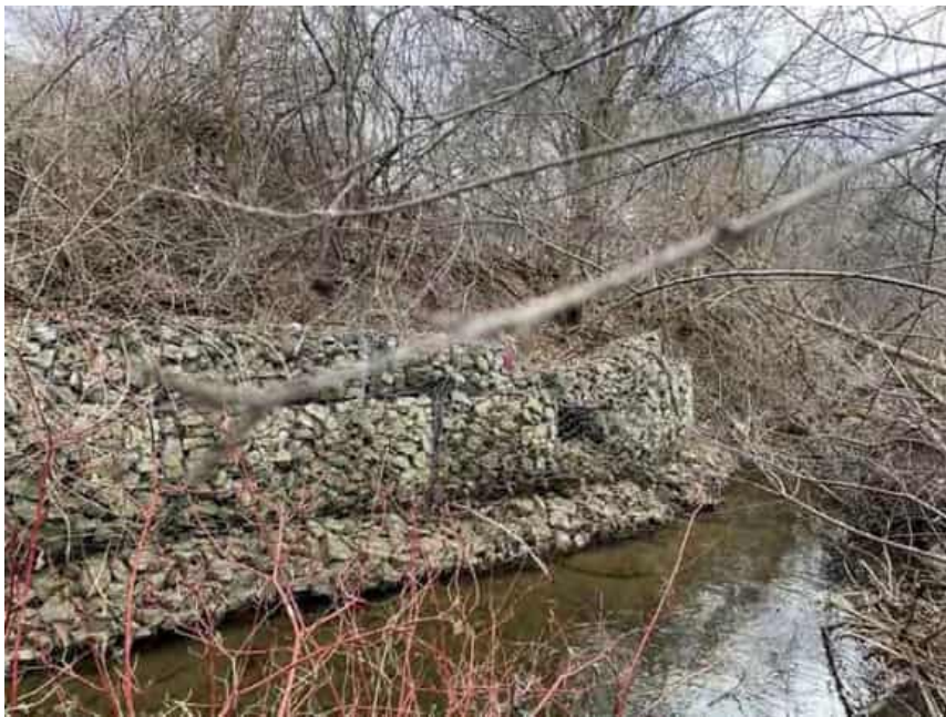
Photo 16: Gabion baskets along the east bank of reach 3
