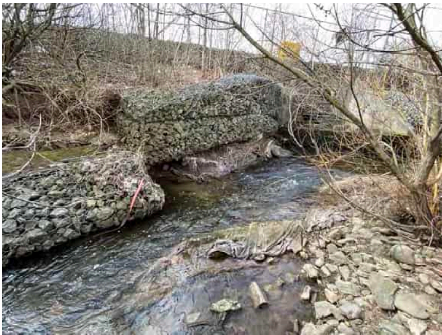
Photo 14: Gabion baskets along the west bank adjacent to the Appleby GO parking lot stormwater outfall
