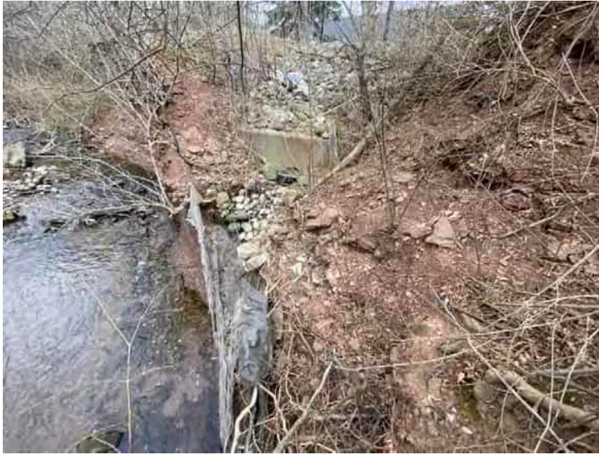
Photo 18: Bank erosion immediately upstream of stormwater outfall adjacent to the parking area of Branthaven Homes
