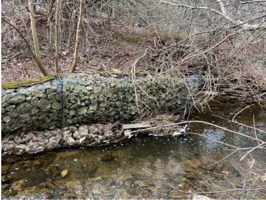
Photo 14: Gabion baskets along the west bank adjacent to the Appleby GO parking lot stormwater outfall
