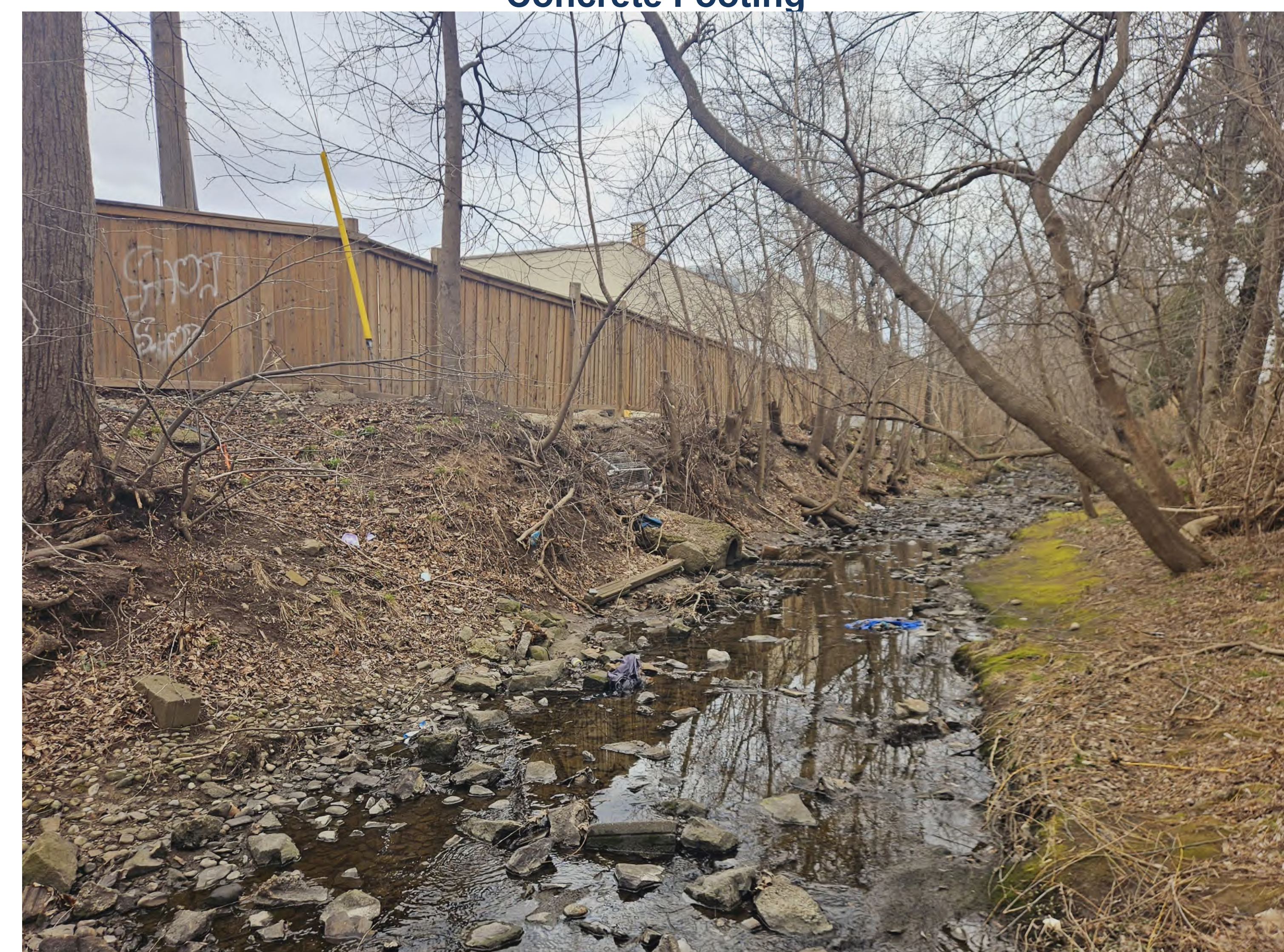
Photo F – Looking Upstream – Shallow Stream Bed and Leaning Tree
