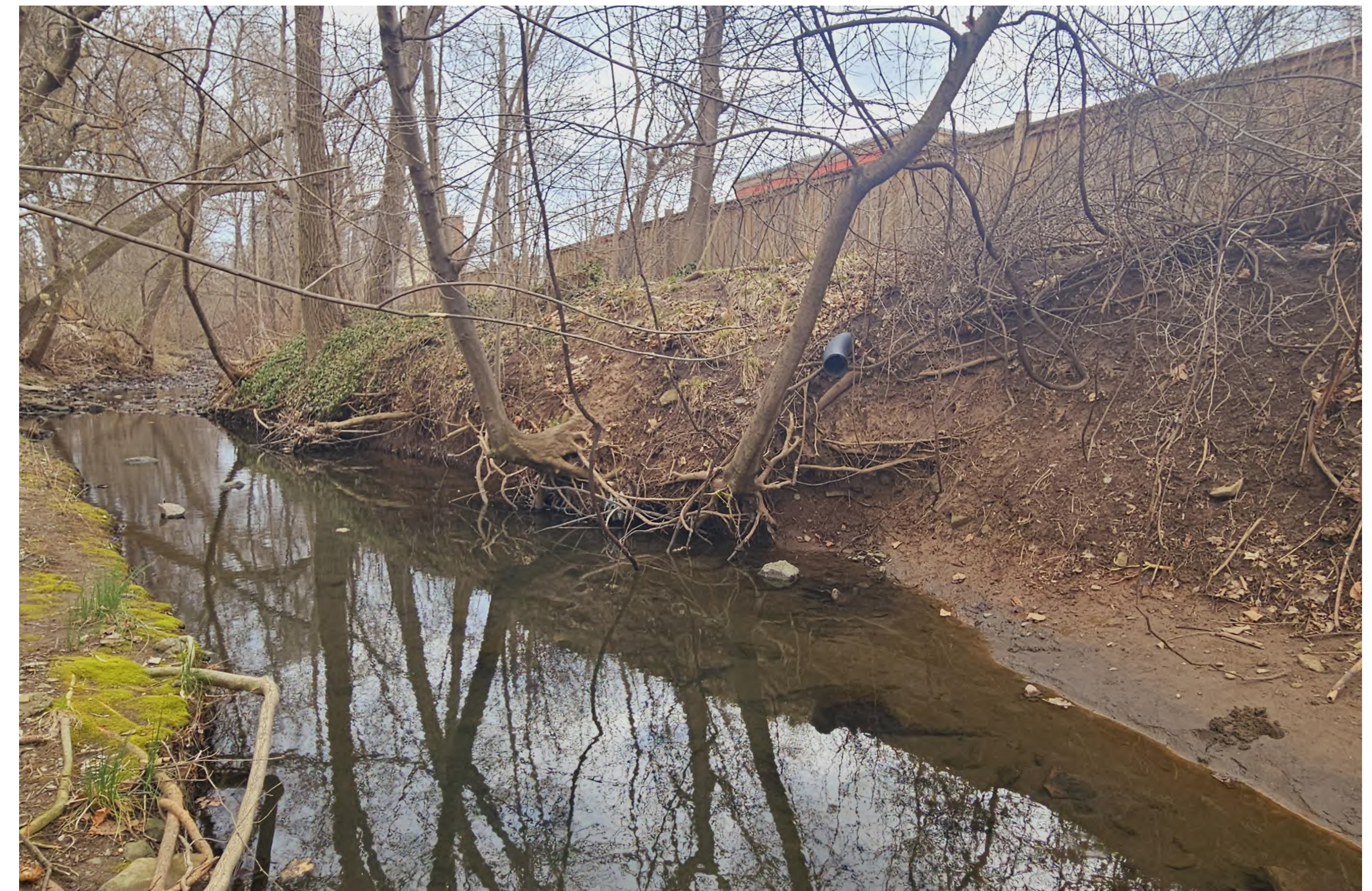
Photo A – Over Steepened Unstable Bank and Overhanging Trees
