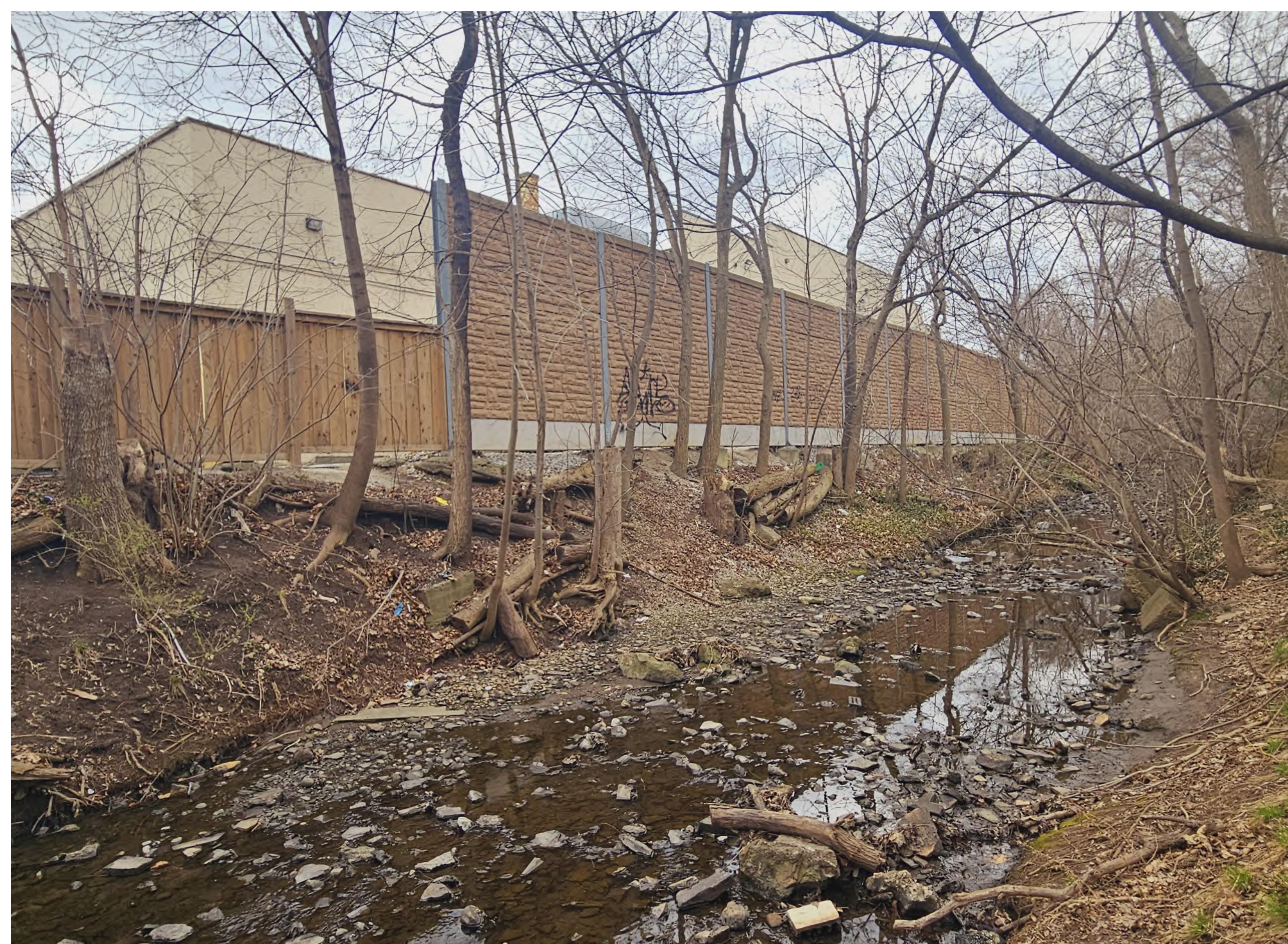
Photo E – Close Proximity of Wooden Fence and Concrete Wall Situated on Top of the Steep West Bank
