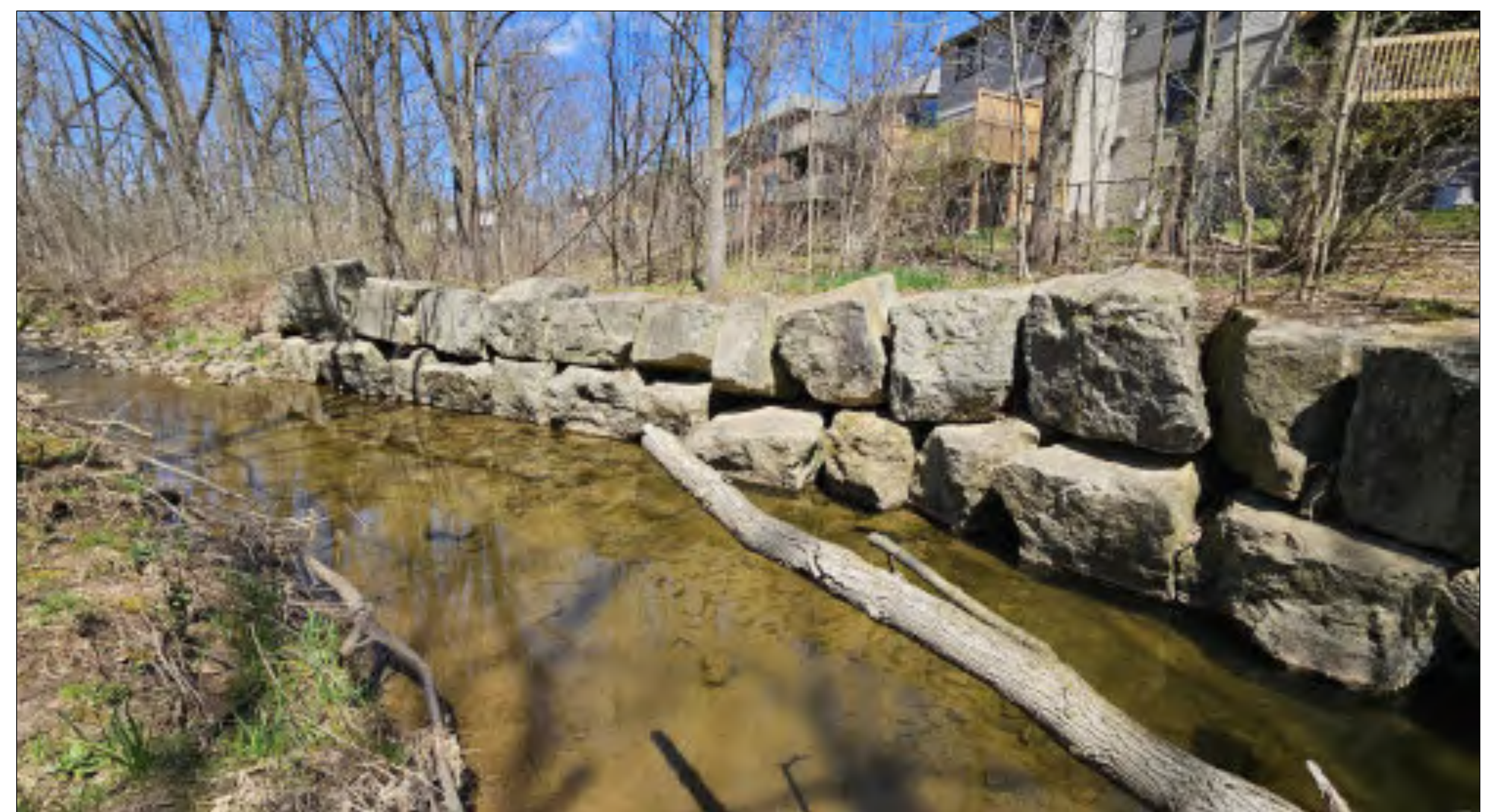
Photo C – Armourstone Wall in a Deteriorated Condition
