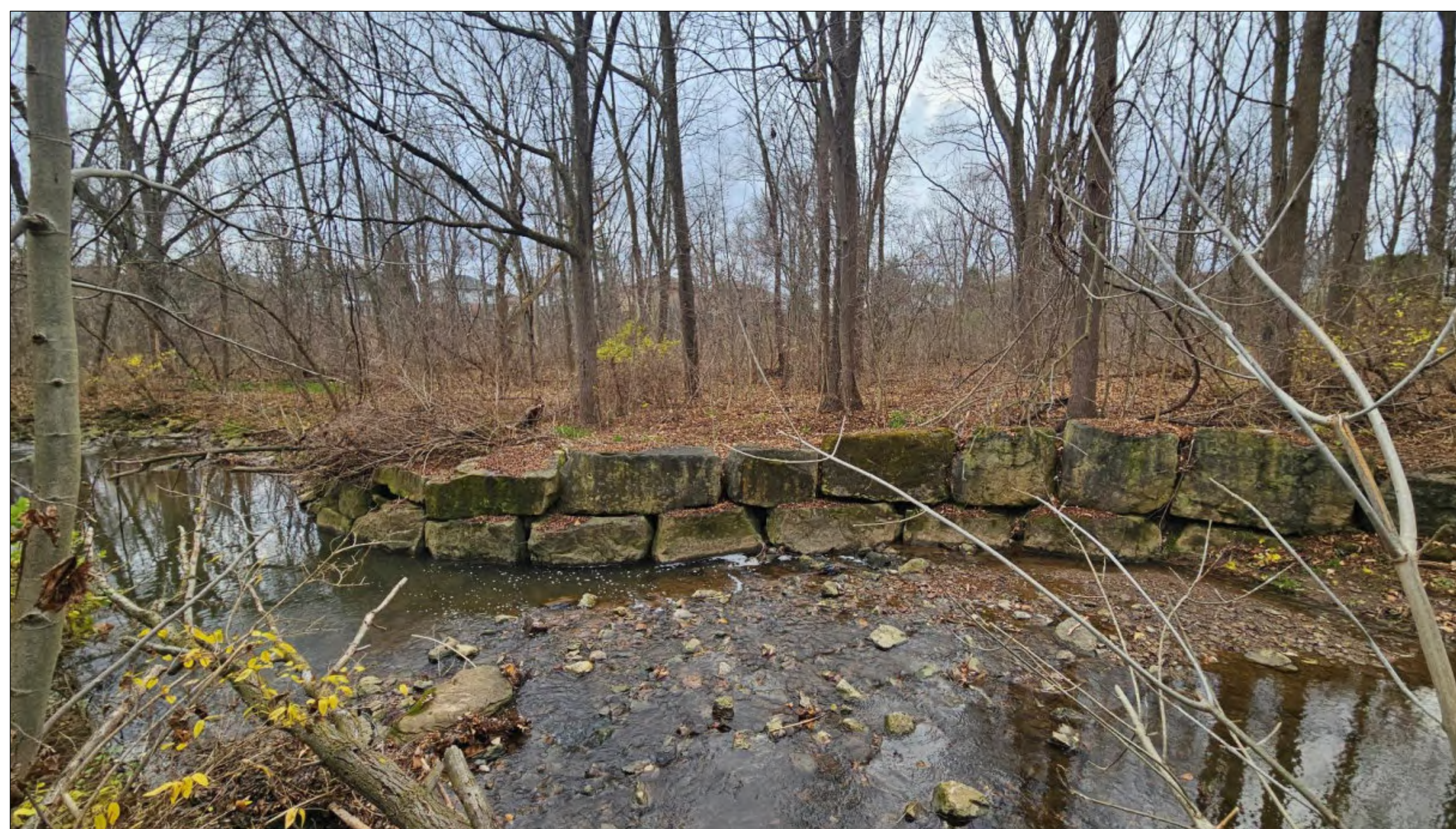
Photo B – Failing Retaining Wall Falling Towards the Creek
