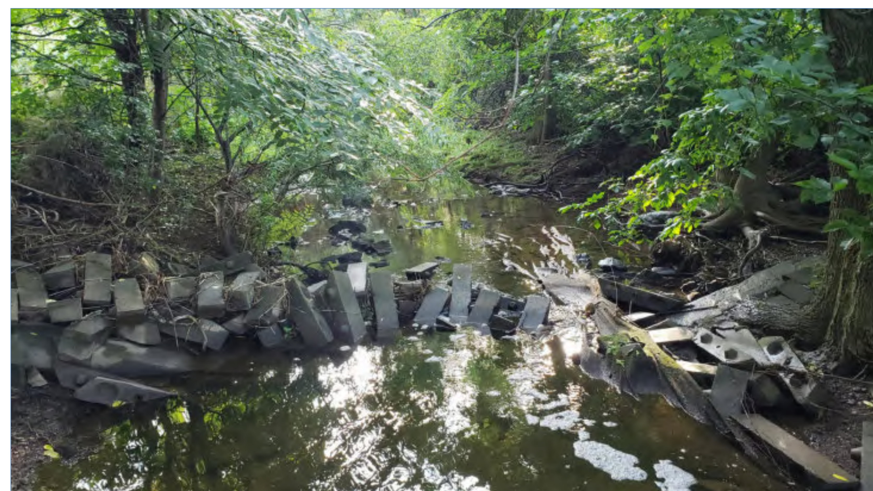
Photo C – Failed Terrafix Blocks Downstream of Concrete Weir
