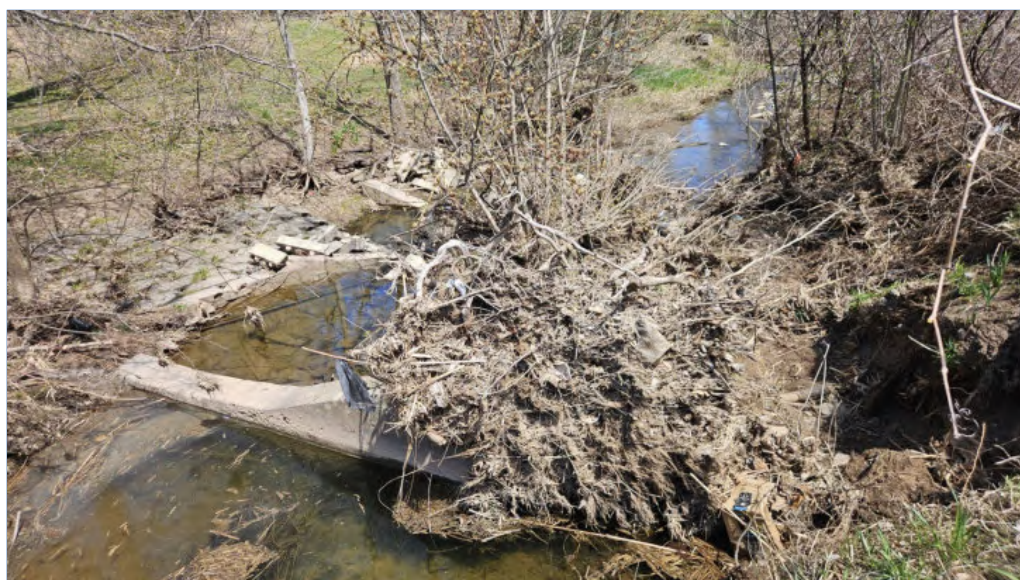
Photo B – Outflanked Concrete Weir with Downstream Terrafix Blocks Lining Channel
