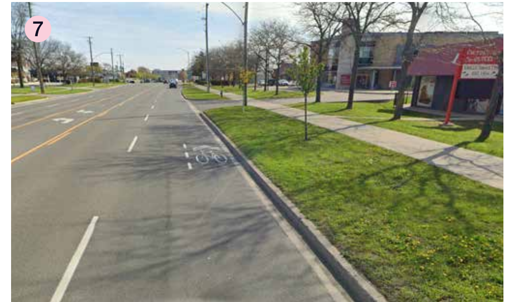
Dedicated Bike Lane on Fairview Street
