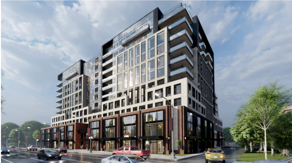
Front of building
