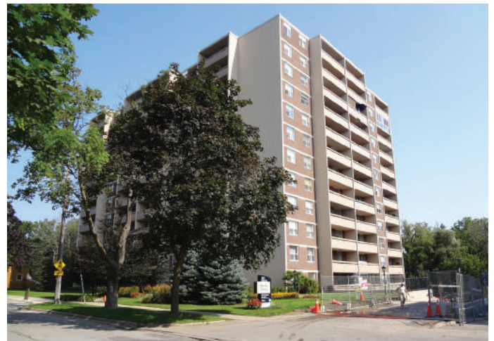
Martha Terrace Apartments, existing tall building in the 'tower-in-the-park' style.
