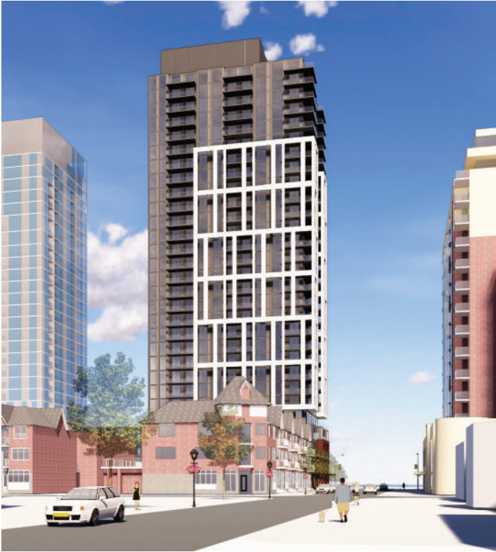
Rendering of the original proposal looking southeast from the intersection of Pearl Street and Pine Street. Note the distinct characteristics of the podium and tower, and the ways in which the tower is articulated, using balcony style and position to add visual interest.
