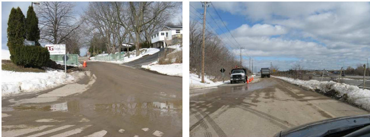
Feb 15, 2013 – Even without rain, mud from construction vehicles tracked all the way to Waterdown Road from Panin Rd. This may also happen on Waterdown Road with construction vehicles exiting and could become hazardous to motorists.
