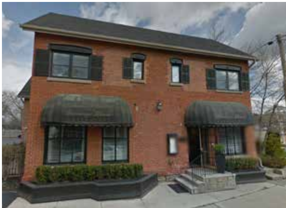
9) 2101 Old Lakeshore Road (Google Maps).
